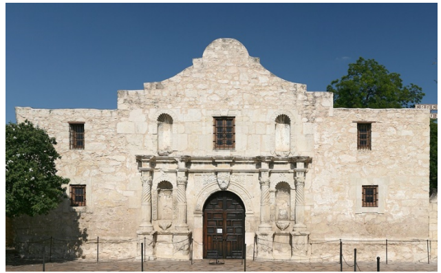
The Alamo, San Antonio, TX
